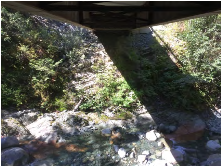
Left Bank Abutment when facing downstream
