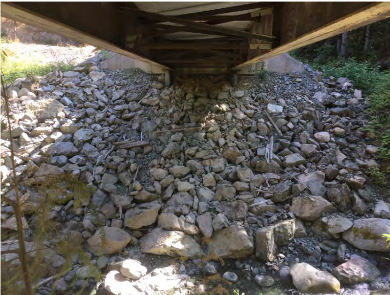
Right Bank Abutment when facing downstream
