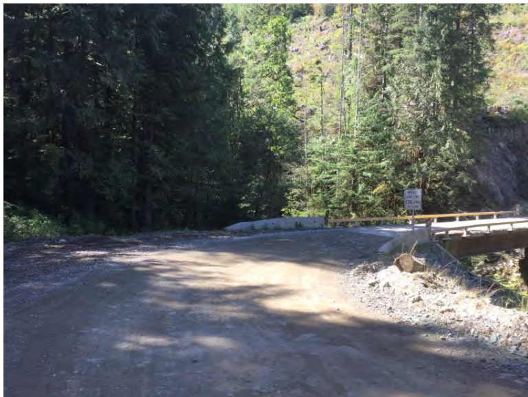
Approach from Right Bank when facing downstream
